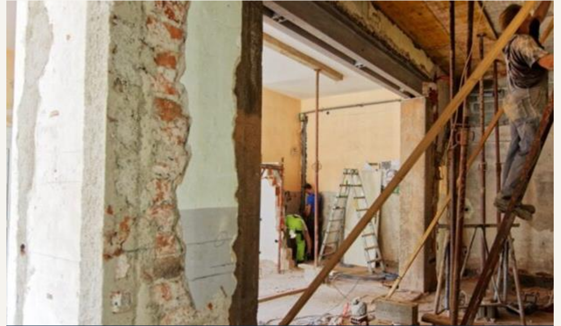
Renovation and repair work
